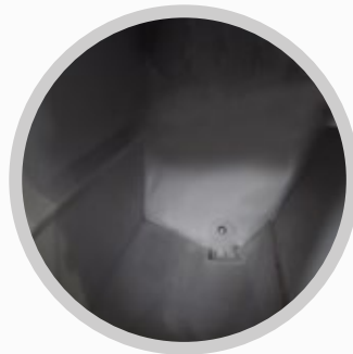
SLOPED TANK BOTTOM WITH LOW DIPPED DRAIN
